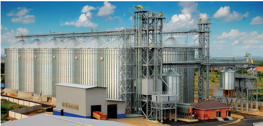
Figure 1. Modern grain elevator
