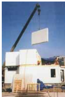
Fig. 6. Building assembling using large panel directly from the transportation truck.
